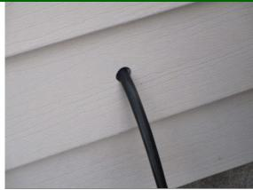
Exterior Surface: Unsealed entry into siding.
